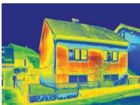
Thermal Image of Condominiums
